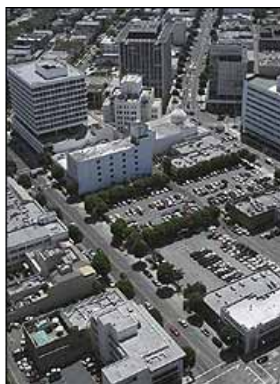
The hotel will be built in a part of Beverly Hills, Calif., known as the Golden Triangle.
